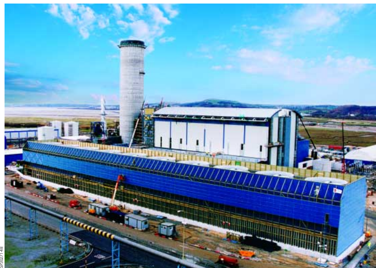
Baglan Bay power station is the launch site for GE's H System ™.
