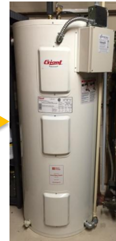
1 st completed tank installed, Les Crittenden
