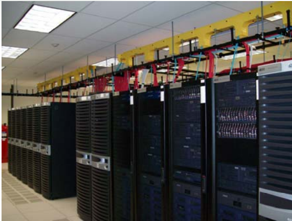
Accessible equipment racks with overhead cable trays
