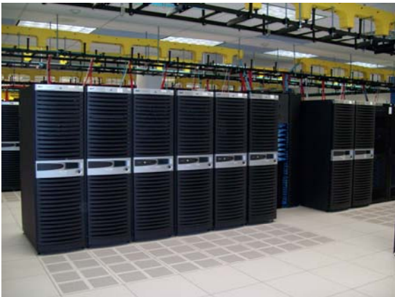
Accessible equipment racks with overhead cable trays
