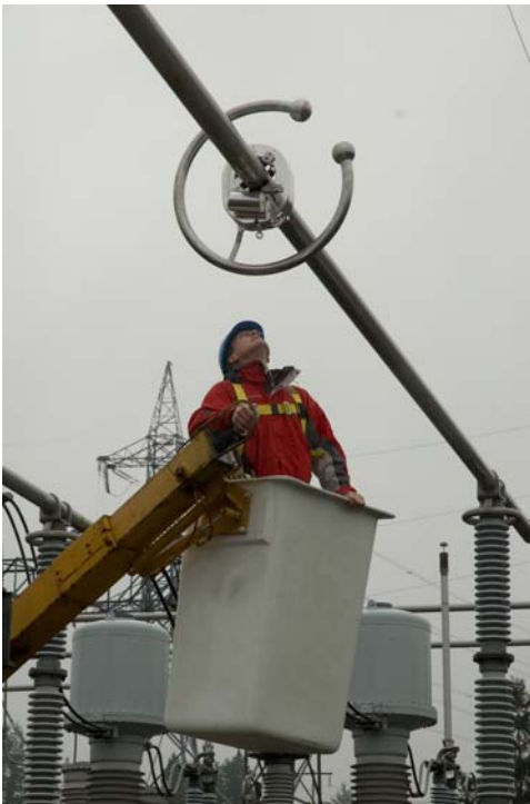
Figure 8 (left) installing the Battery Powered Primary Sensor
