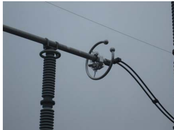
Figure2. Self-power HV Primary Sensor (left) and Figure 3, the Battery Powered Primary Sensor (above)
