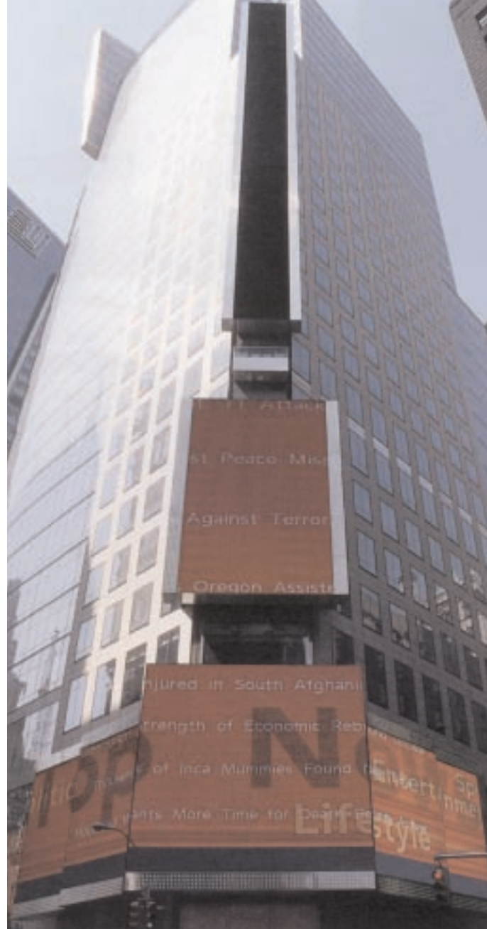
As energy markets become more competitive, consumers are more aware of finite power resources, and the need to conserve. The Reuters Building, at 3 Times Square, is "smart, green, and ready," consuming 30 percent less energy than similar office buildings. Owner Rudin Management accomplished this by using more natural light, glazing external glass to deflect sunlight from entering the interior of the building, as well as state-of-the-art motors and fuel systems in the heating and ventilation network.
