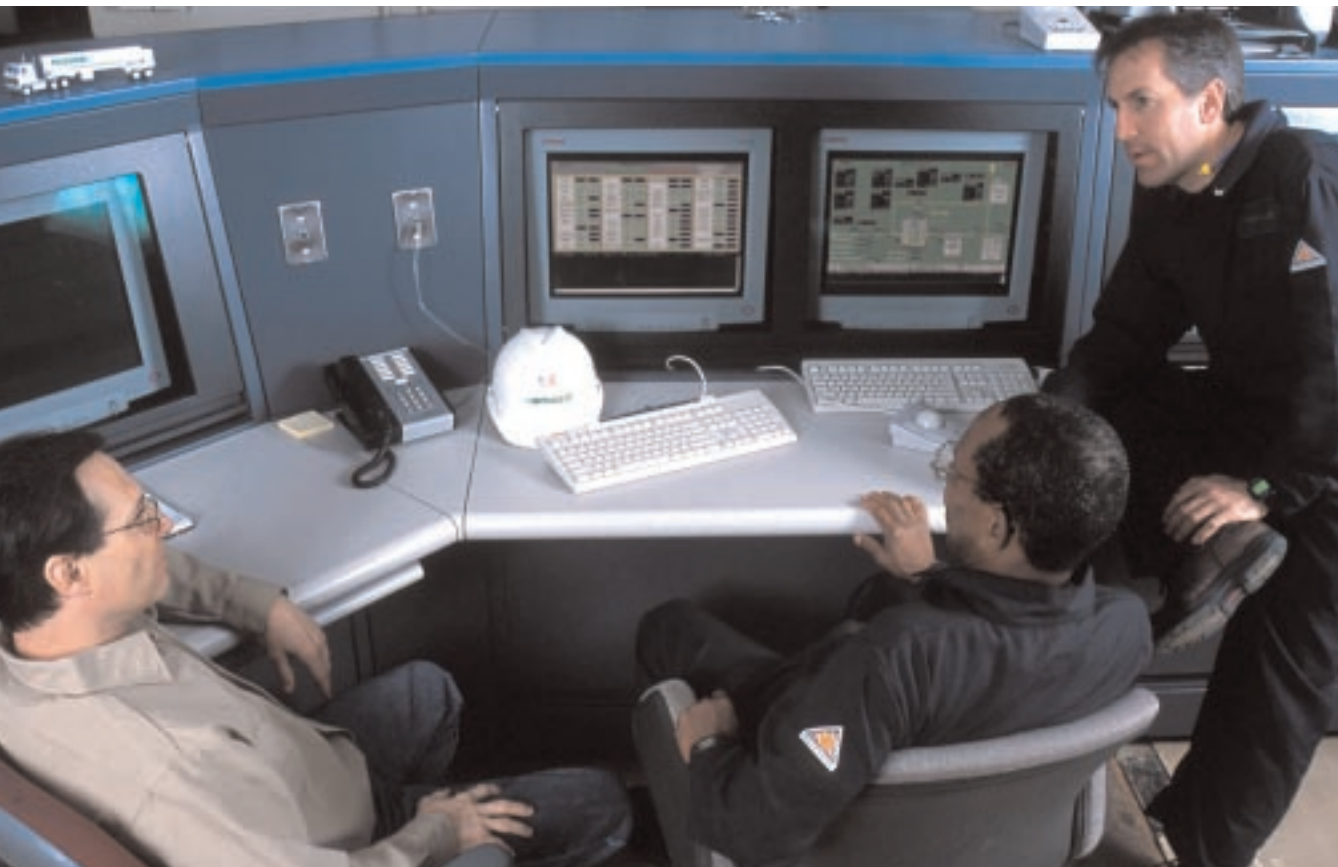
Production Technicians Eddy Jeanty and Chuck Barone confer with Plant Manager Christian Lenci at Praxair's production facility in Niagara Falls. The facility's new computer control system was installed in May 2002 and funded in part by payments from the NYISO's Emergency Demand Response Program (EDRP). "During times of extremely high electricity demand, Praxair turns its plant off so other New Yorkers can keep their lights on," said Lenci. "The NYISO has developed one of the best demand-response programs in the country; Praxair is proud to help out when the NYISO needs it most."
