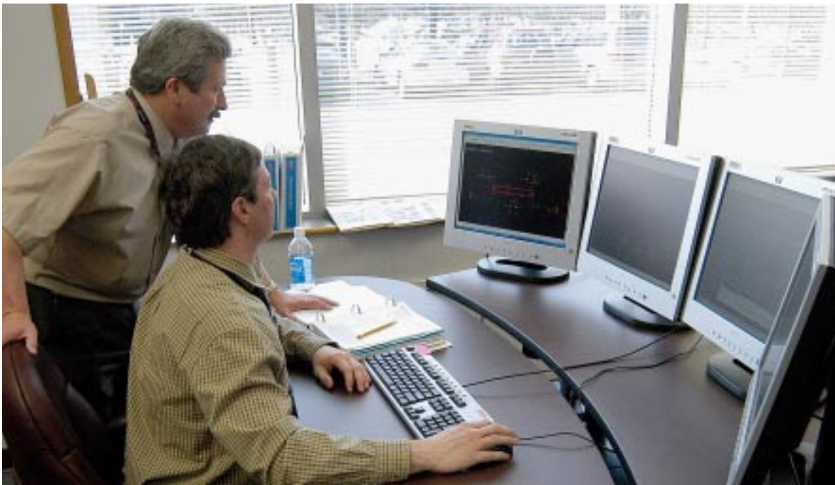
NYISO grid operators annually receive four times the amount of training recommended by the North American Electric Reliability Council. Pictured are Control Center Shift Supervisor Mike Egan, standing, and Robert Shellhouse, dispatcher.
